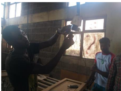
SCH electrician Temesgegn “in action”
